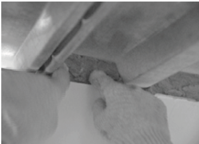
Figure 2. Installing filler material.
