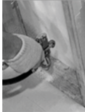
Figure 6. 3500SI can be installed by spraying or with a brush or roller.
