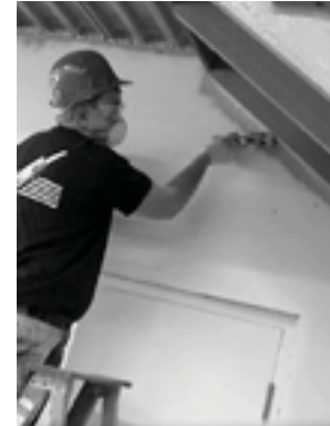
Figure 6. 3500SI can be installed by spraying or with a brush or roller.
