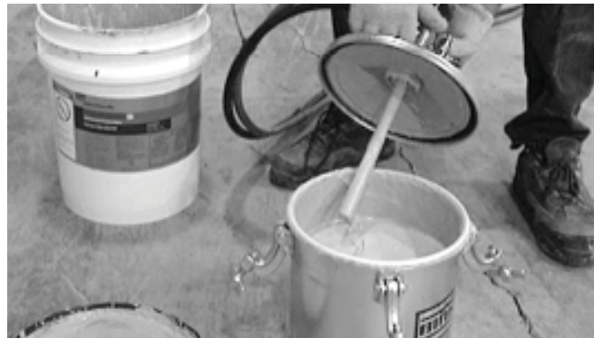
Figure 3. Pressure pot with 3500SI spray ready to be closed and pressurized.
